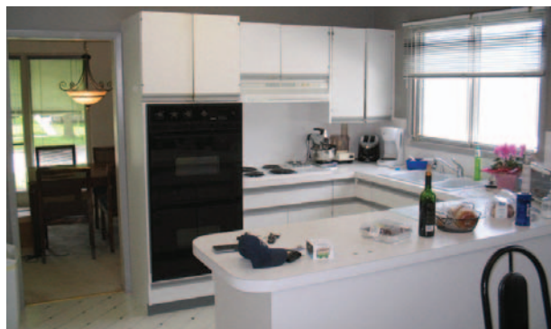
The “crunched” kitchen before All Canadian Renovations’ transformation.
